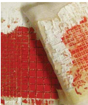
(Separation of plaster)
